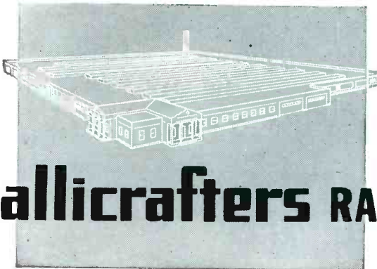
HALLICRAFTERS NEW $600,000 HOME NOW UNDER CONSTRUCTION.
